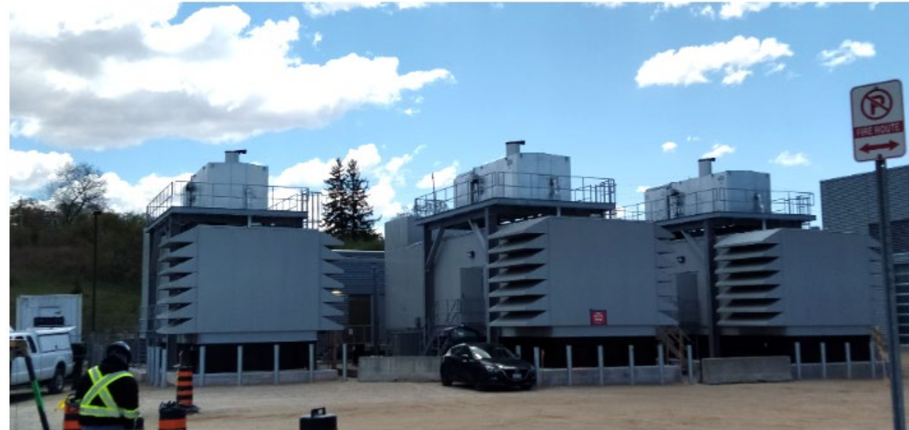
Image: Tier 4F equivalent retrofit on a Tier 2 generator. Steel pillars would be installed on either side of the enclosure supporting a platform and a walkway around the unit.
